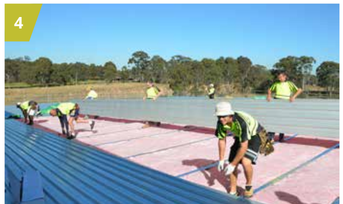
4 Roof Razor® is wide and stable enough to walk and balance on.
