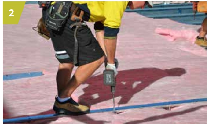
2 Roof Razor® spans the entire blanket width allowing for a direct line of sight to the purlin.
