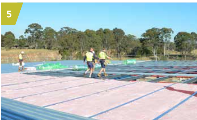
5 Roof Razor® can be comfortably trafficked the same way as a purlin.
