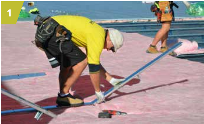
1 An overlapping tab specifies where to position the consecutive Roof Razor®.
