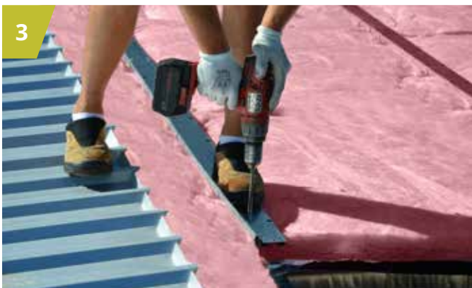
3 Fasteners are pre-loaded and provide easy access to the fastener head.
